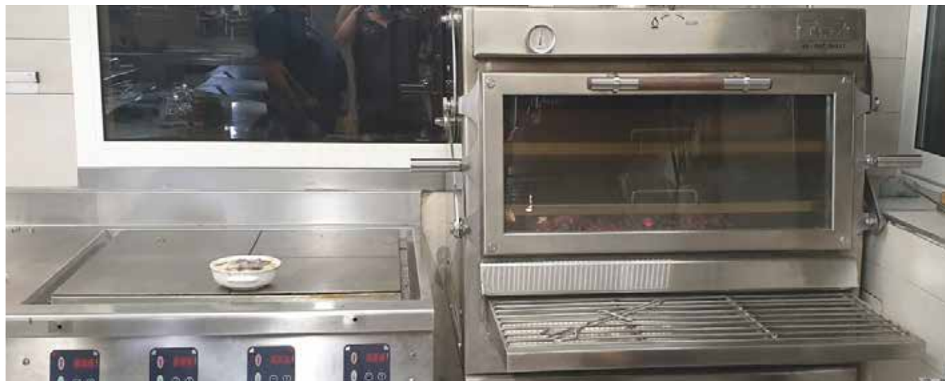
Kitchen detail Restaurant Foier des Guides in Valtourneche (Italian Alps)
