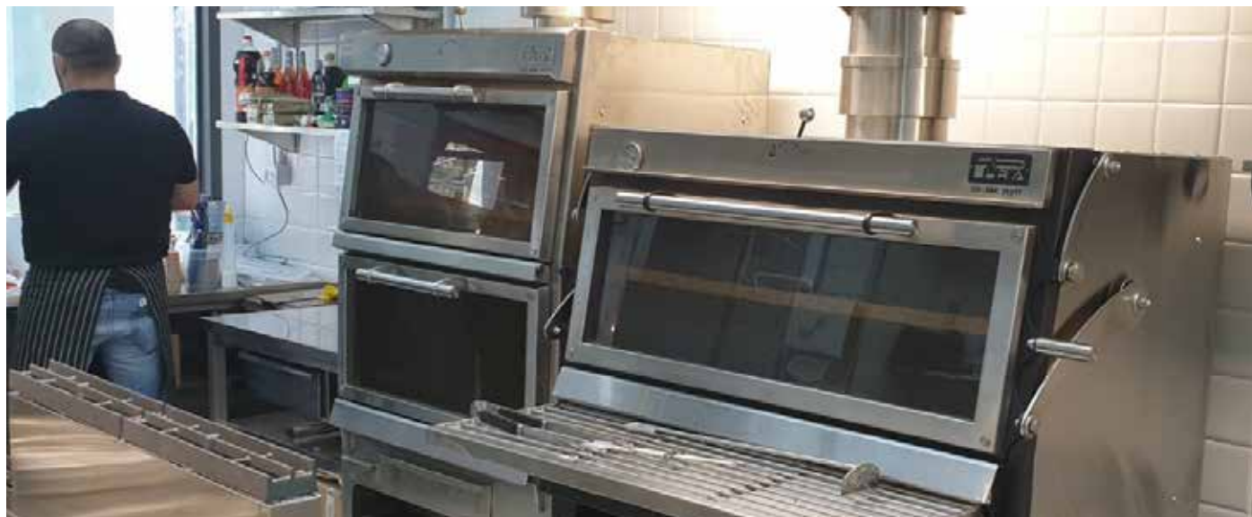
Ara Bracis Restaurant kitchen detail in Rome
